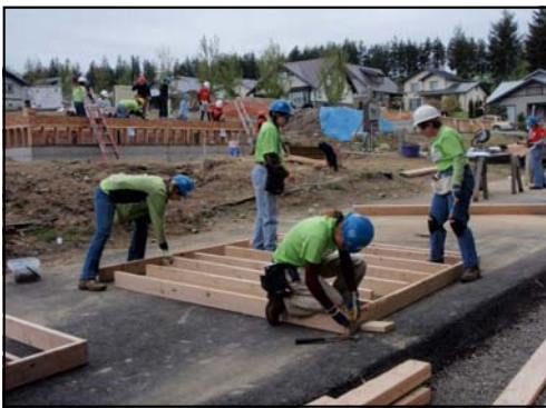
Women Build Volunteers frame a wall.
